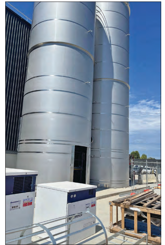
Two 100-tonne corn storage silos.
