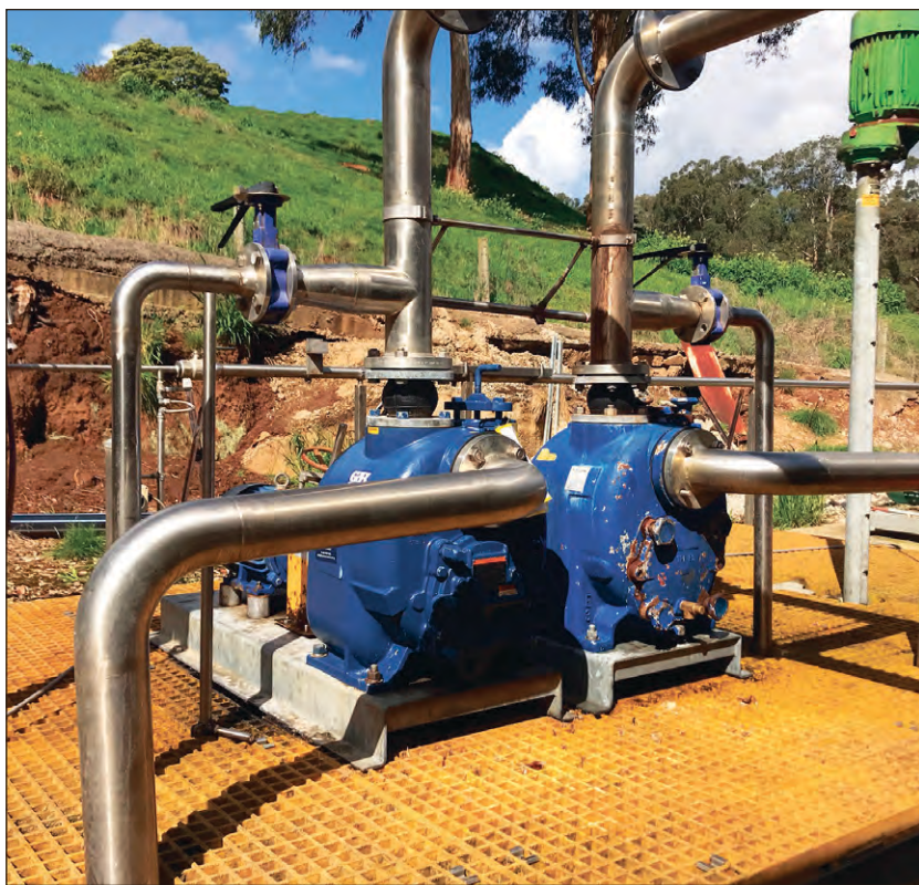
The solution to Central Agri's Trafalgar plant wastewater pump issues was a Gorman Rupp T3A71S-B 'Super T Series' trash pump fitted with an 'Eradicator' solids management system.
