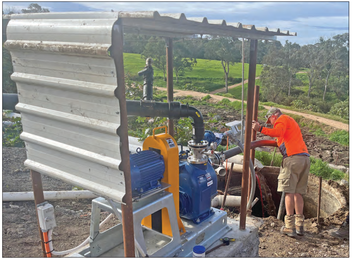
Within a day of operation, the Gorman Rupp Super T3C60SC-B, fitted with the solids management system, had waste material pumping steadily to the separator screen.
