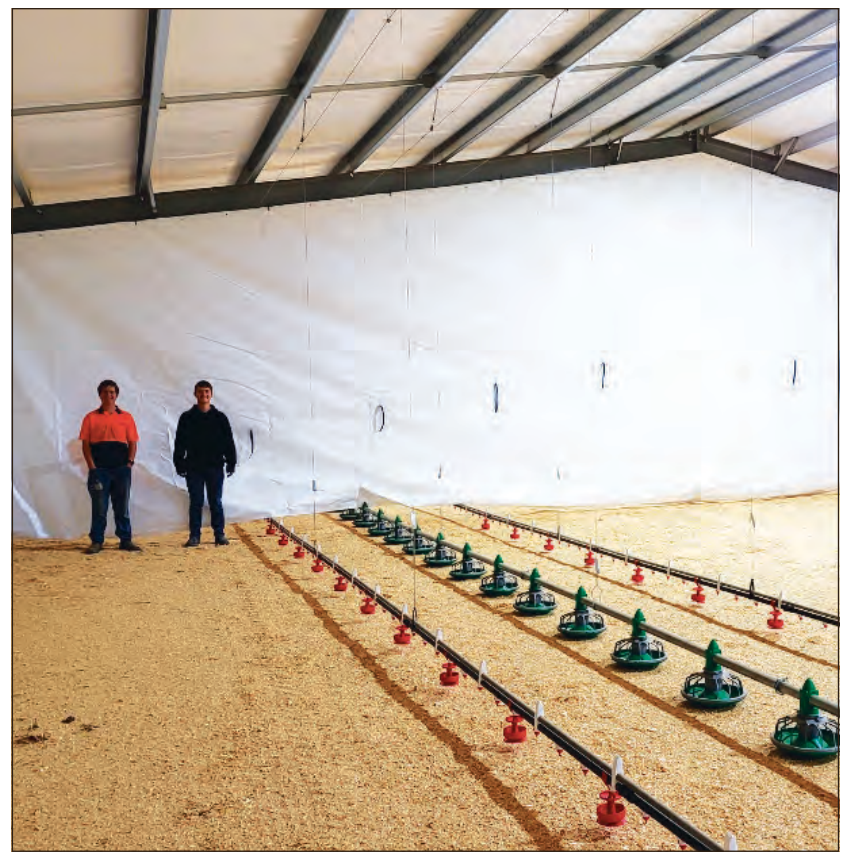
Poultry shed brooder curtains provide more efficient energy usage.
