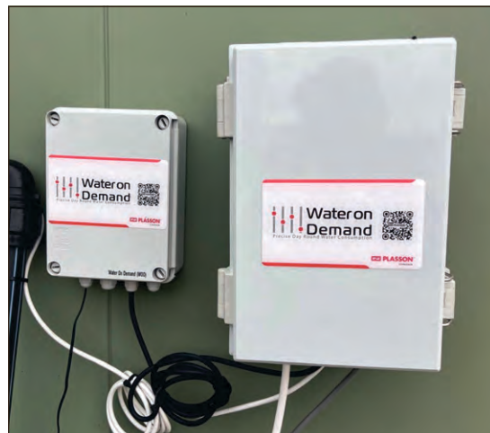
Technologies such as 'Water On Demand' enable producers to automatically adjust water pressure profiles throughout the day.
