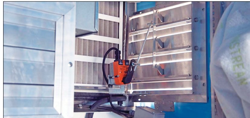
Carbon dioxide is contained within healthy levels, via automated opening and closing of fan-assisted vents. So ambient air is mixed at the AC outlet collector as required.
