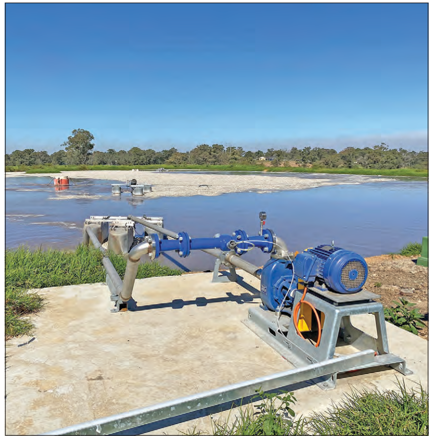
Venturi aerators reduce odours at AJ Bush & Sons.
