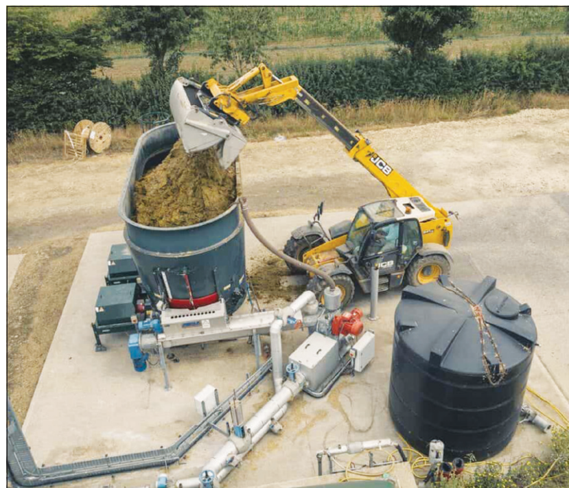
An anaerobic digester is like a concrete cow stomach. Materials are fed into the digester, broken down by bacteria and converted into methane.
