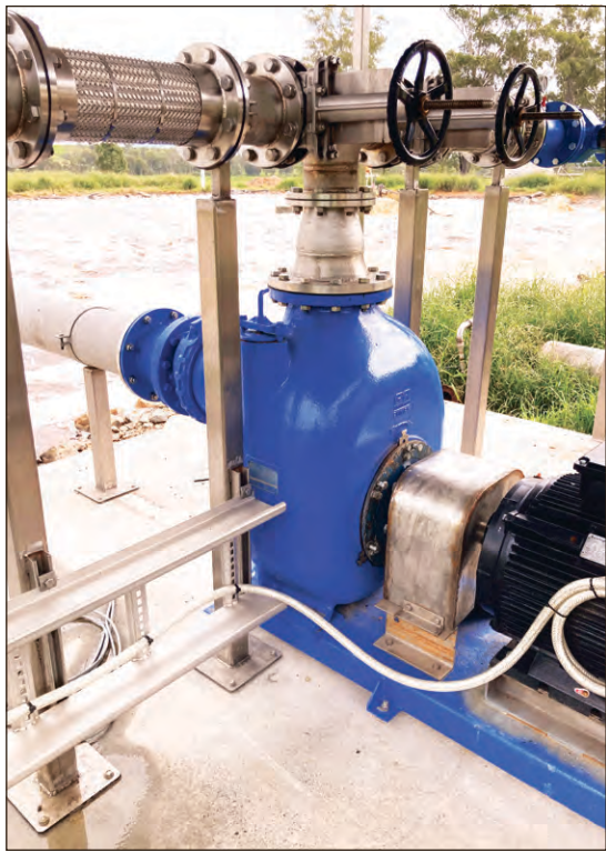
Gorman-Rupp 'Super T Series' self-priming wastewater pumps are easily accessible for monitoring and maintenance.
